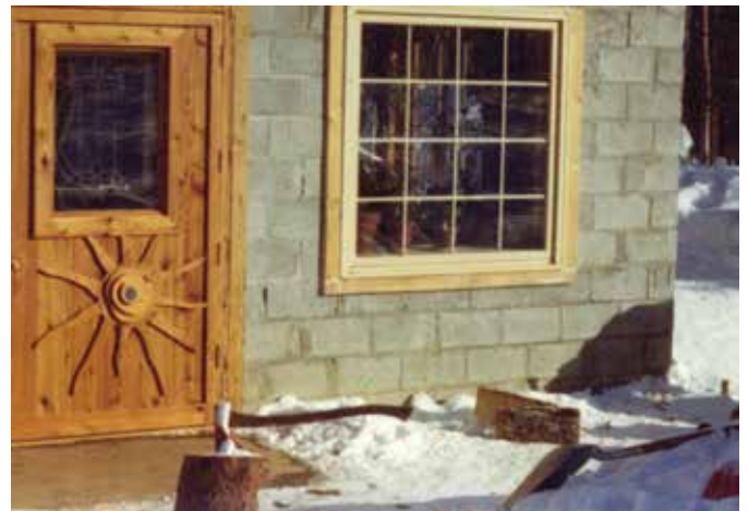
Front door with a thermal protective cover for the stained glass door window. Photograph: Robert Roggasch
