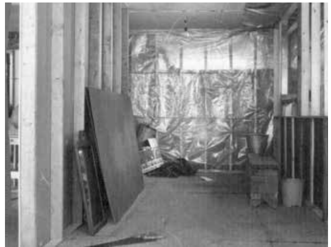
Bedroom image shows a one third/ two third thermally broken vapor barrier wall system. Refer to the Canadian R-2000 for similar systems. Photograph: Robert Roggasch
