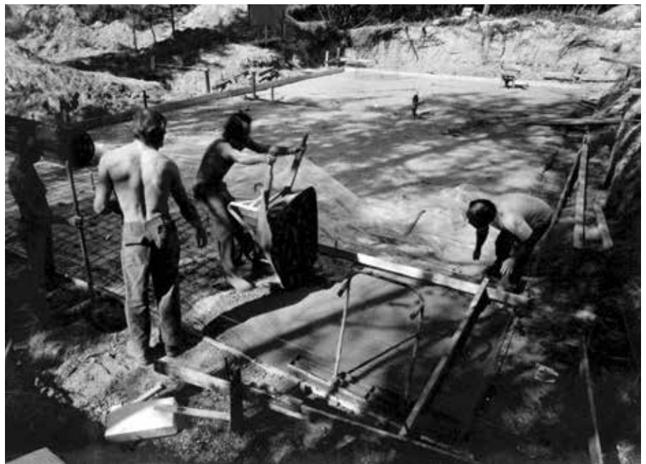
Pouring the concrete slab with friends. Photograph: Ann Roggasch.
